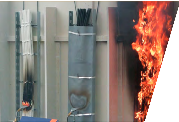
Comparative fire behaviour of cable trays (from left to right)
